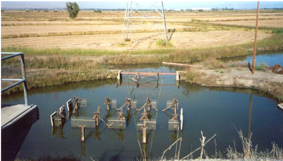
Figure 13. Photograph of old Pumping Plant No. 3 sump and toe drain (looking northeast).
