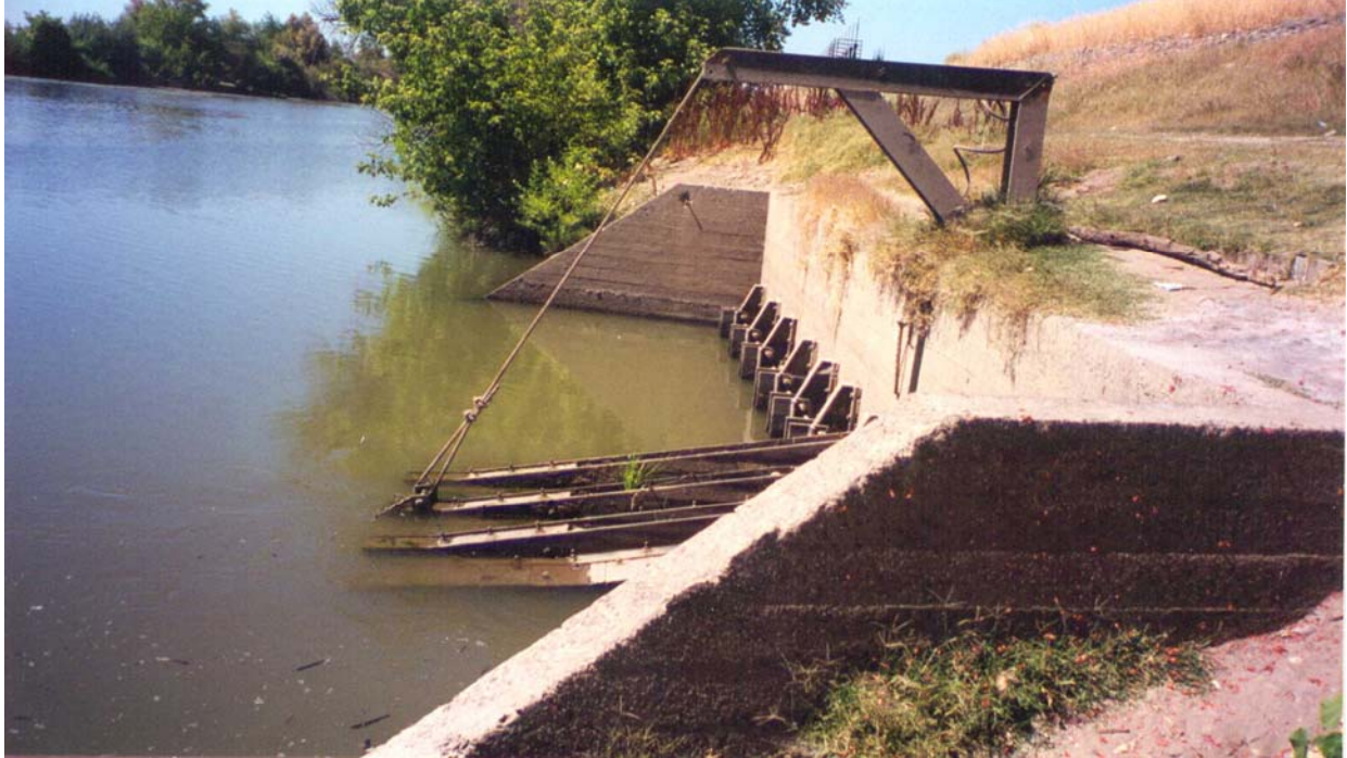
Figure 11. Photograph of headwall structure and flap gates (looking upstream in the EBC).
