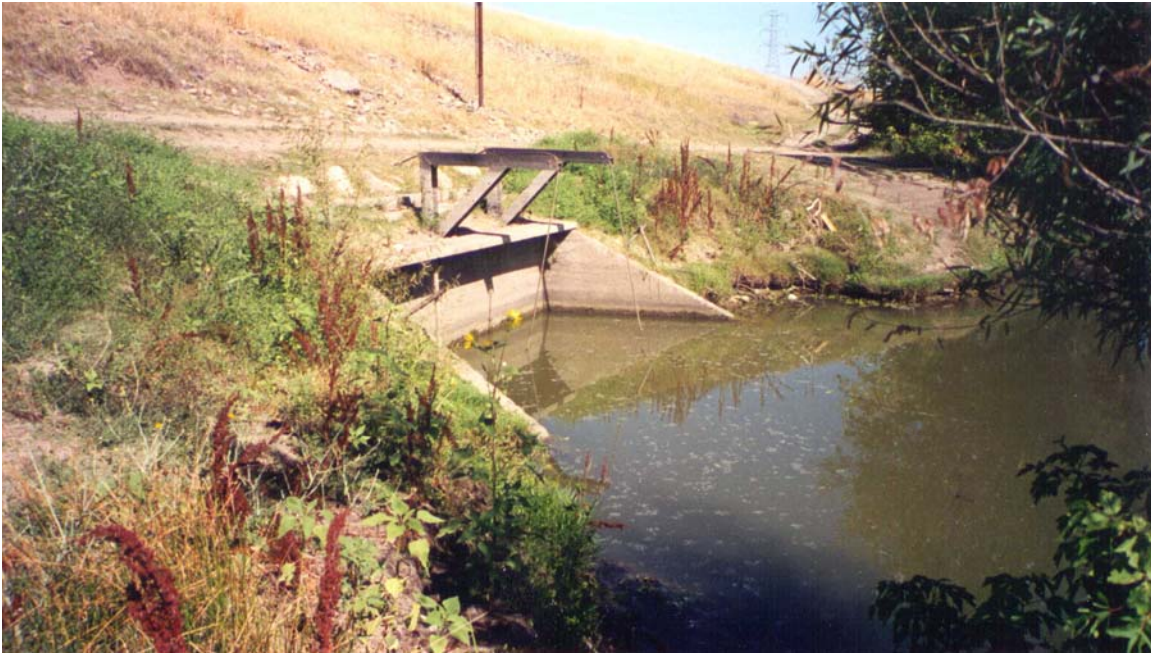
Figure 7. Photograph of headwall structure and submerged flap gates (looking downstream of EBC).
