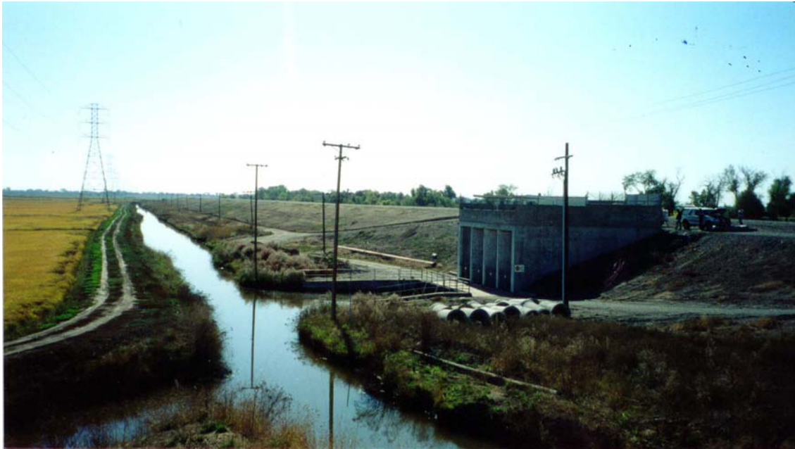
Figure 6. Photograph of new Pumping Plant No. 1 and south toe drain (looking south).
