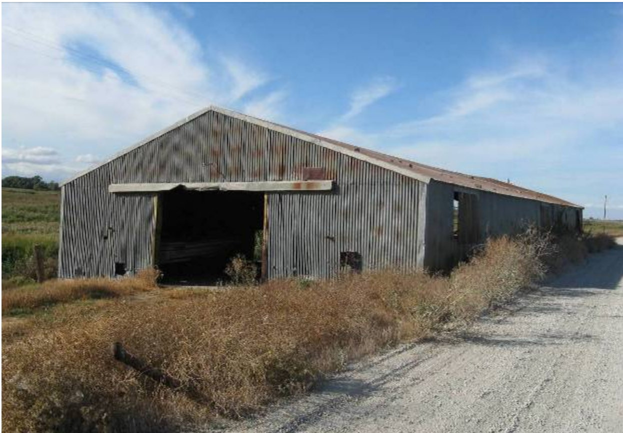
Figure 4.6-3 Soulé Building, looking north
