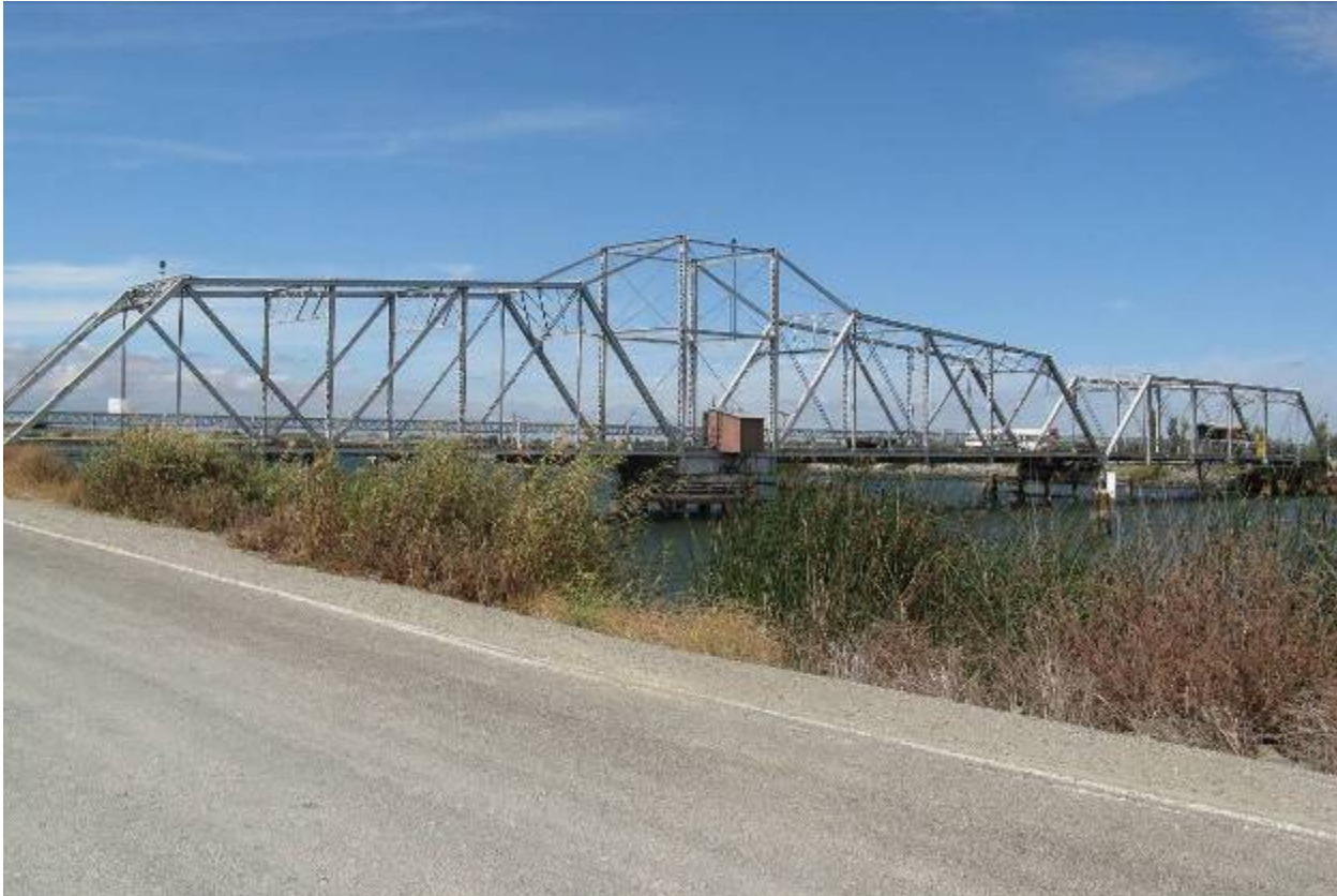
Figure 4.6-1 Truss Bridge across Connection Slough, looking northwest
