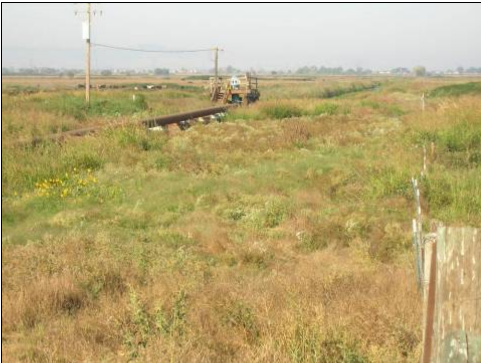
Figure I-3. West bank of the Old River, diked canal perpendicular to the levee road.
