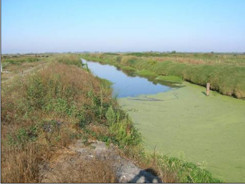
Figure I-4. West bank of Old River, view of diked canal.
