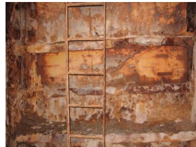
Figure 12. Severe Corrosion near Hatches
