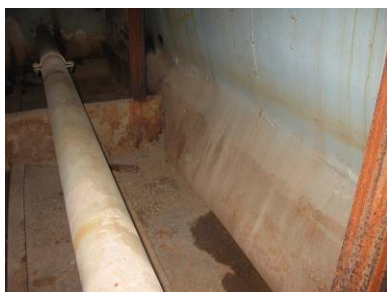
Figure 9. Buckled Bulkhead
