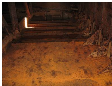
Figure 14. Bottom Patch Plate
