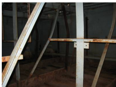
Figure 8. Buckled Stanchions
