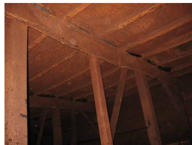
Figure 3. Typical Deck Frames & Stiffeners
