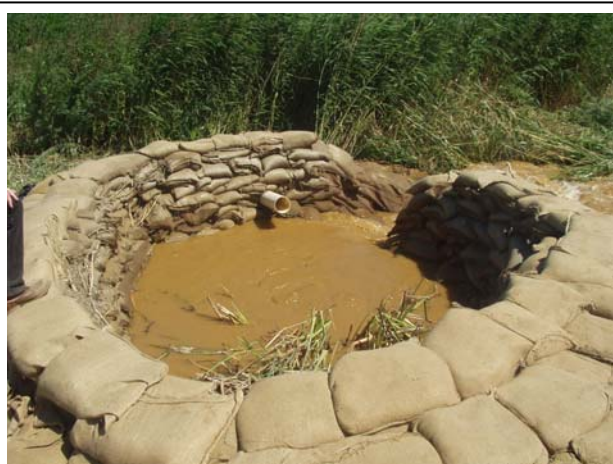
Boil on landside levee bench, Staten Island, Delta (Jul. 2007)
