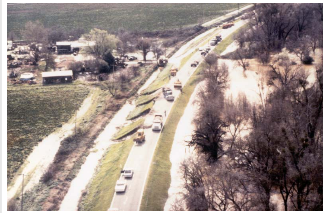
Picture of Sacramento River Levee Through-Seepage failure (USACE 1986) Soil particles were observed moving down the landside slope while water was oozing from the slope face.
