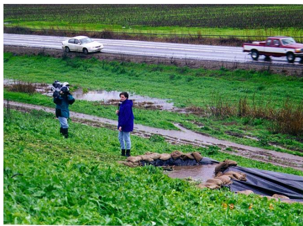
Boil on landside slope, Bouldin Island, Delta (Feb. 1983)
