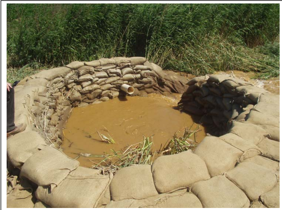
Picture of sand boil at Staten Island (ejecting ~250 gpm) during the near levee failure 6-21-2007 (Picture by DWR 6-21-2007)
