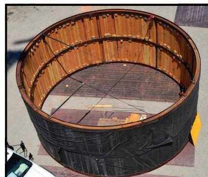
Double steel ring with wood lagging that will be installed at every 5-ft of excavation.
