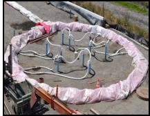
Close-up: Installation of freezing pipes 128 feet down into the ground to form the Newark retrieval shaft.
