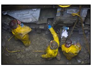
View into the retrieval shaft: Tunnel boring machine breaking through. Crews preparing to cut it for its removal.
