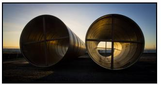
40-ft X 9-ft diameter steel pipe spools part of the 5 mile pipeline connecting the East Bay to Peninsula Bay Division Pipelines.
