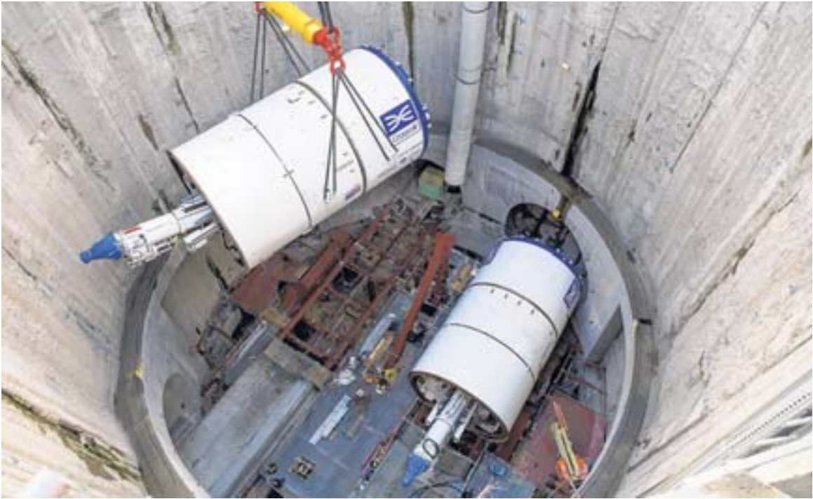
Boring machines for London's new Crossrail rail link are digging 13-mile-long tunnels that cross beneath the city center.
