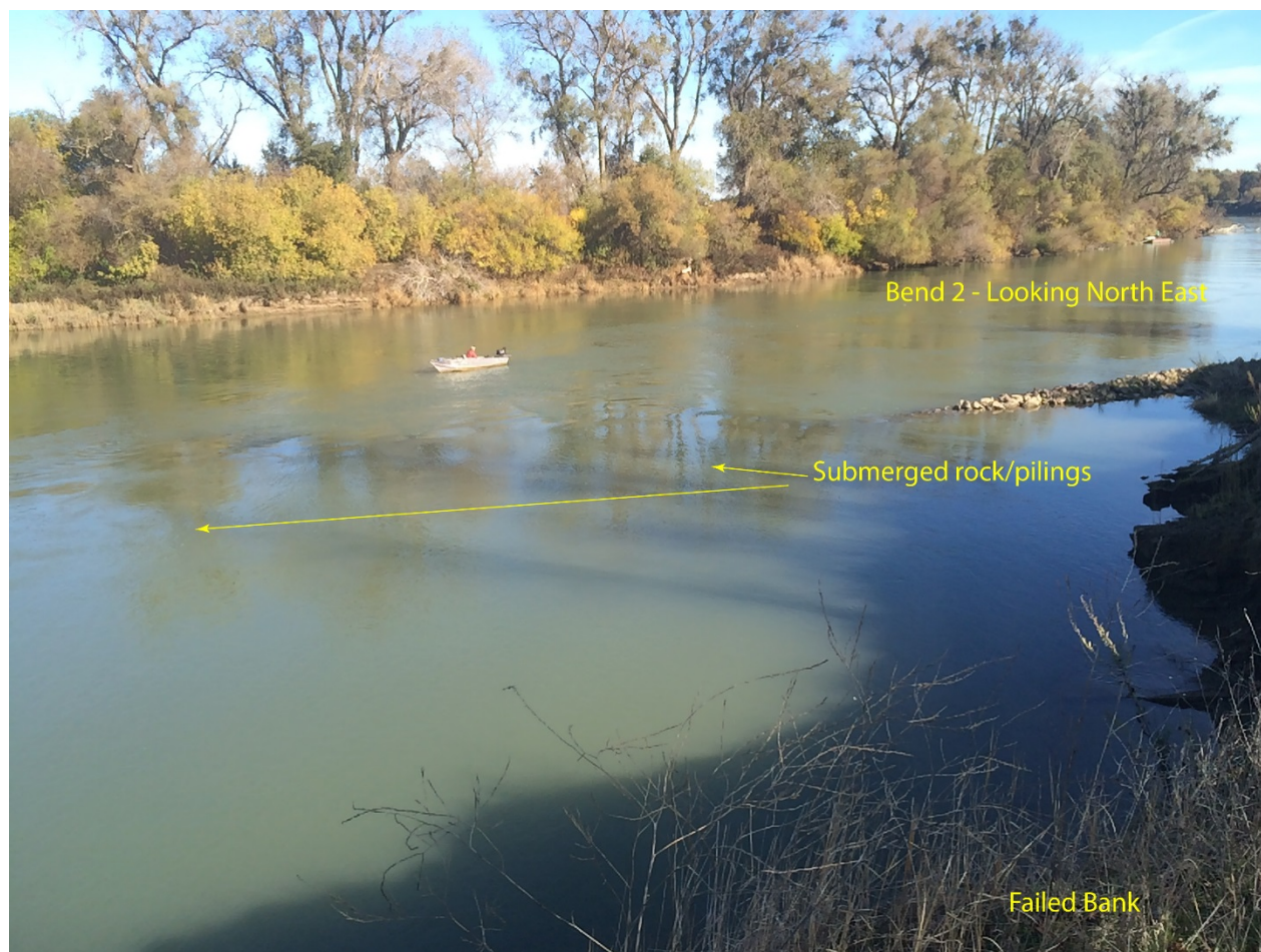
Figure 15 – Photograph of bend #2 taken from the outside of the bend where the bank protection failed looking northeast.
