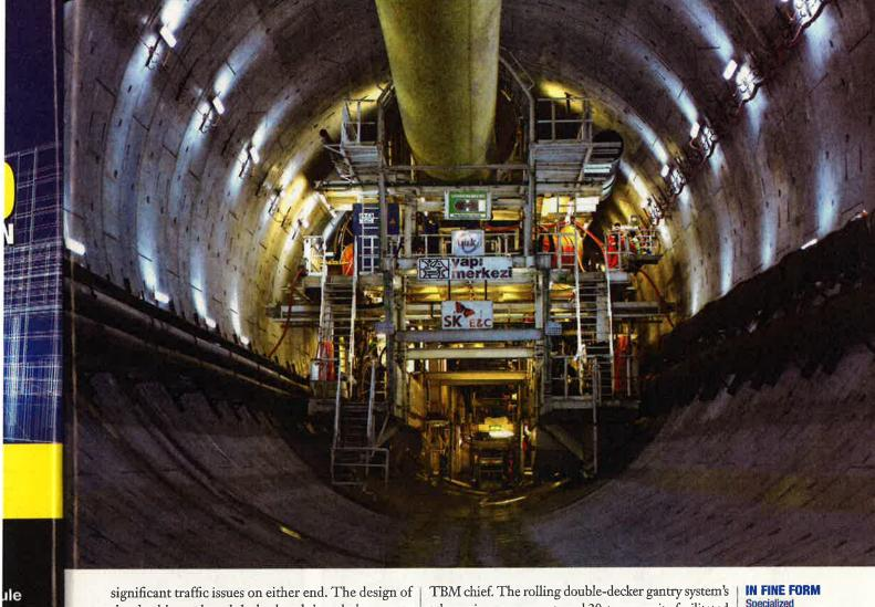
significant traffic issues on either end. The design of the double-gasketed, bolted and doweled precastconcrete tunnel lining, with each tunnel ring consisting of nine 600-mm-thick segments, "is to ensure that this tunnel stays safe and dry," Clarke says.
