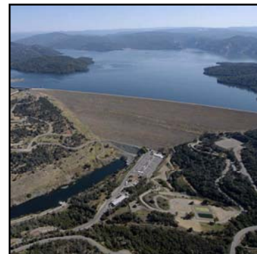
Oroville Dam is part of the SPFC
