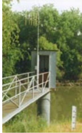
Data collection workstations (satellite and microwave receiver interfaces) are the first piece of the CDEC server network (see The Network diagram other side). They collect data, such as precipitation, stage, and temperature readings, which are transmitted to the microwave and satellite receivers.
