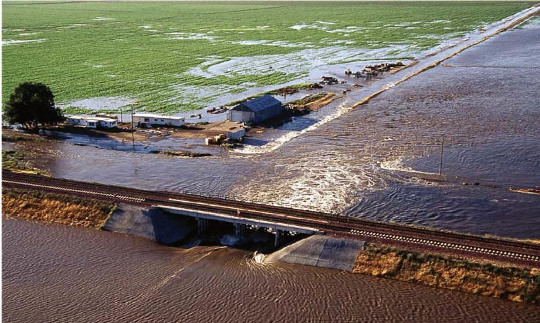
**Figure 1.5 Upper Jones Tract levee breach at noon on June 4, 2004 (photo)**
