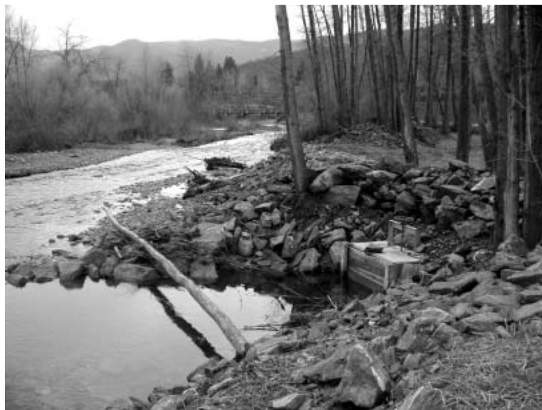
Head gate to a diversion off Shackleford Creek, in the Scott Valley, California, which is a spawning and rearing stream for threatened coho salmon. There is a fish screen just below the head gate, out of the picture.
